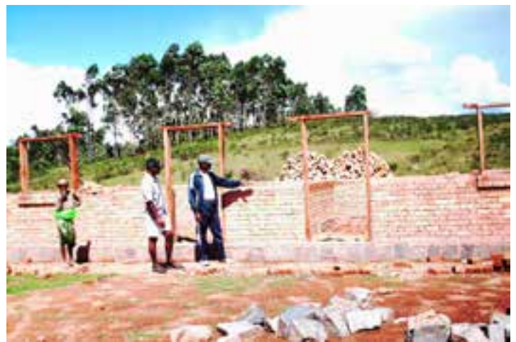
Fig. 3. School construction under progress.
